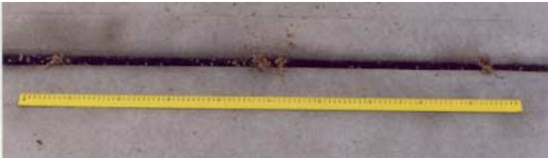
Figures 1, 2 and 3 - Periodic Clustering in Crease between Concrete Slabs
