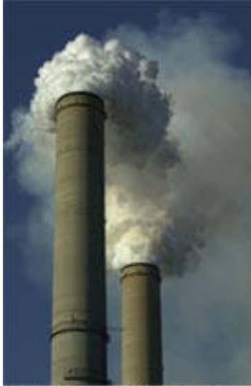
The Gen. J.M. Gavin plant is Ohio's largest coal-fired plant. (Bob DeMay)
