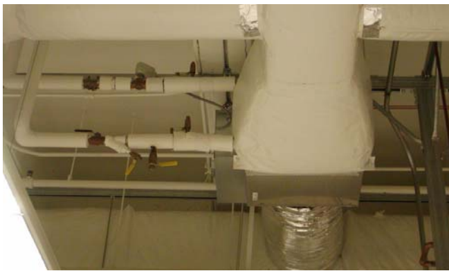
View of Typical Installation and of AVV Assembly
